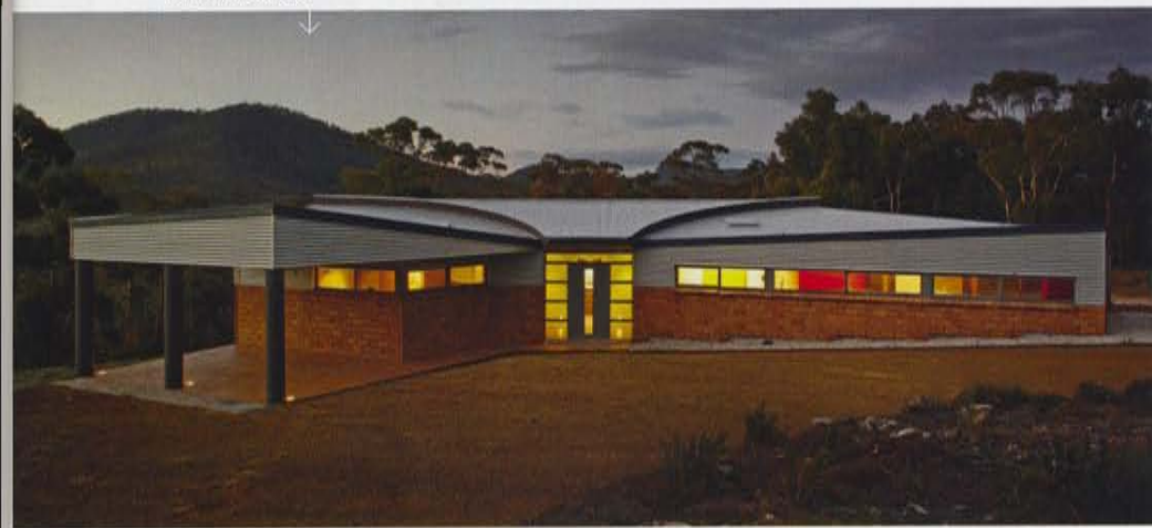
The compressed earth bricks on the southern entry side of house are a striking feature
